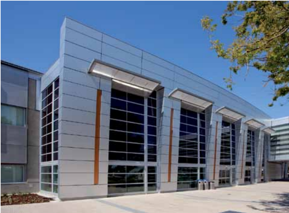
Figure 2: EC glass installed in the Student Services Center at Chabot College, Hayward, CA (exterior view) which is an example of how EC glass can provide additional design freedom to architects. In this case the use of EC glass enabled the use of a natural ventilation system while maintaining a fully glazed south and west facing atrium.
