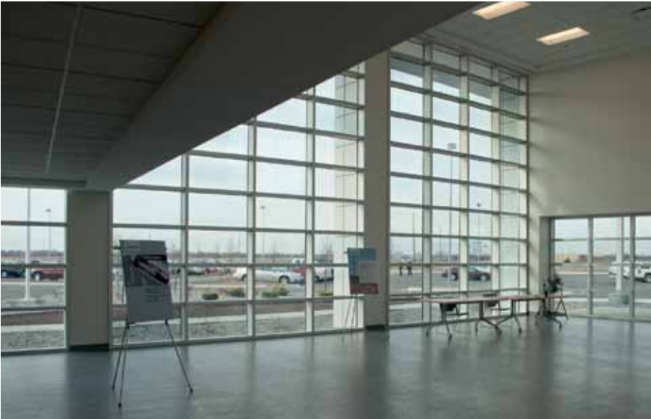
Figure 7: View from the inside of the Siemens Wind Turbine Facility. The EC glass is in the clear state flooding the interior with natural daylight on a cloudy day.
