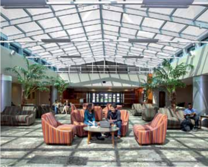
Figure 4: Dehority Hall at Ball State University. A fully EC glazed roof with clerestory encloses a courtyard to provide a multiuse space. This image shows the EC glass in the clear state condition with the clerestory in the fully tinted state.
