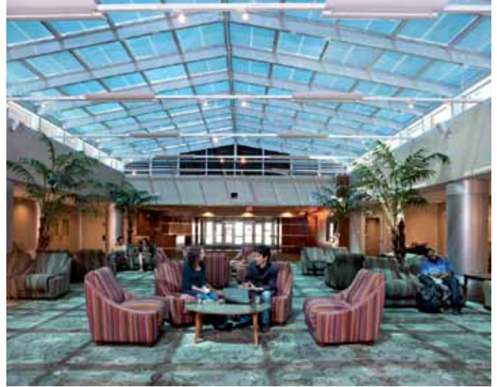
Figure 5: Dehority Hall at Ball State University (as in figure 4). The EC glass is in an intermediate state of transmission between fully clear and fully tinted maintaining a set light level in the space.
