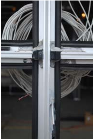
Fig. 4. Holes where the wire is routed into the glazing pocket are grommetted and sealed with silicone.
